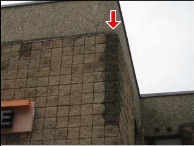
4.0 Item 11(Picture) Flashing joint at corner.
