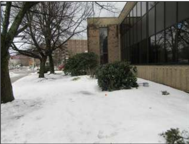
1.0 Item 1(Picture) Right side of building.
