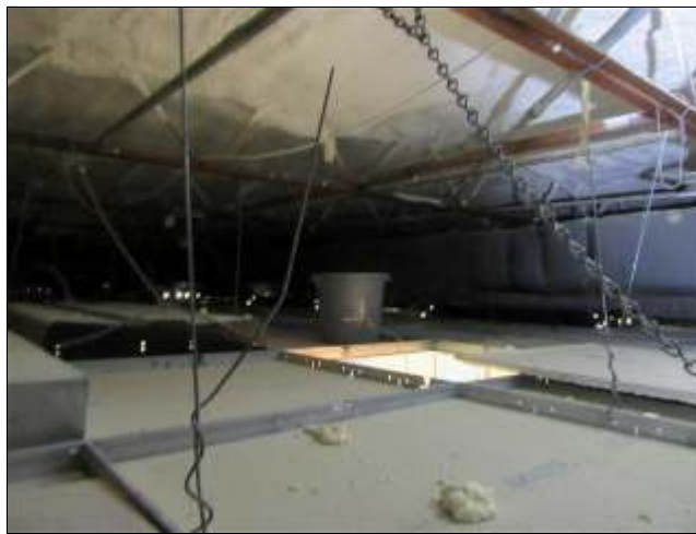
3.5 Item 2(Picture) Roof structure well insulated.
