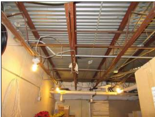
5.2 Item 3(Picture) Floor structure/good condition.
