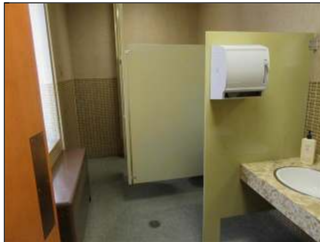
Men's restroom/2ND floor.
