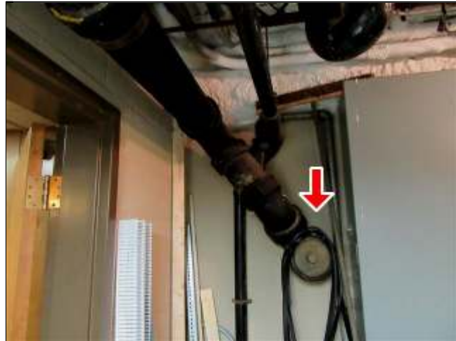
6.4 Item 2(Picture) Storm water drain.
