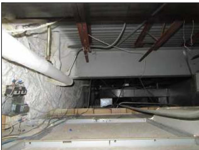
5.4 Item 3(Picture) View of perimeter insulation.
