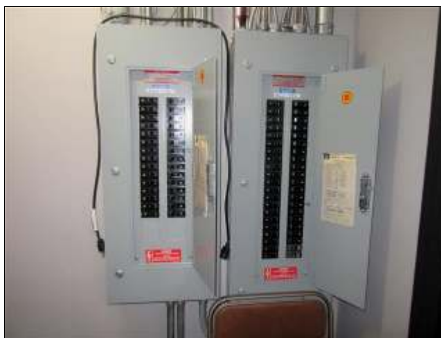
7.1 Item 4(Picture) 2ND floor panels.
