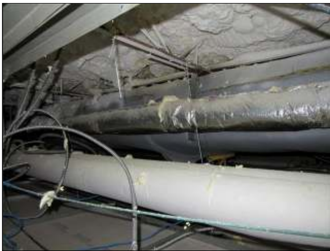
3.5 Item 1(Picture) Typical spray foam application.
