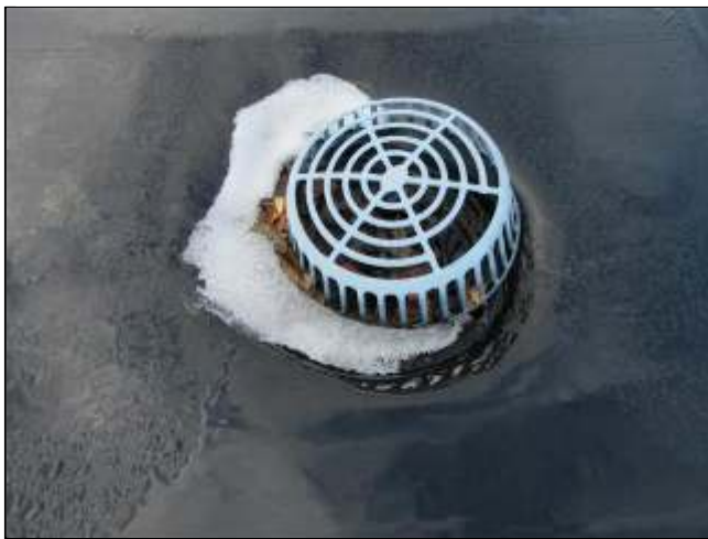
3.3 Item 1(Picture) Roof drain/typical.
