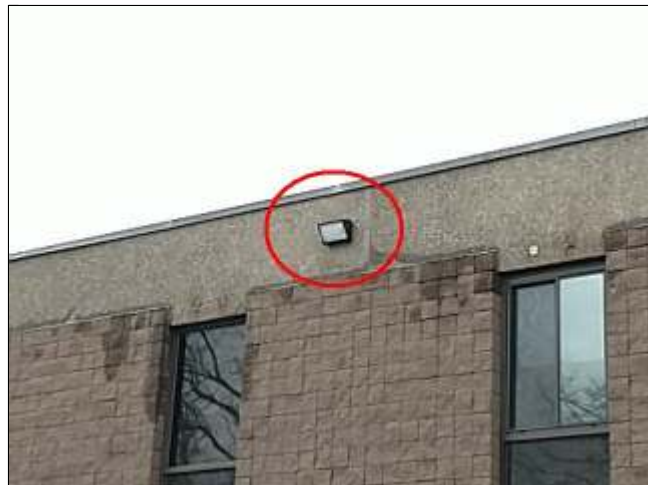
1.4 Item 2(Picture) Typical surface mounted light.
