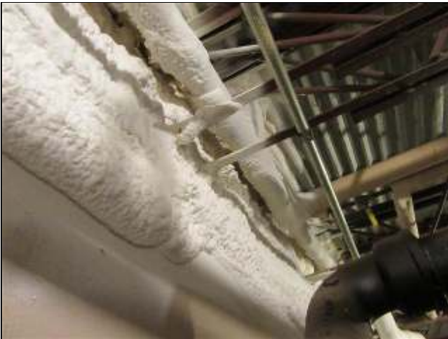
5.2 Item 1(Picture) View of open web joists.
