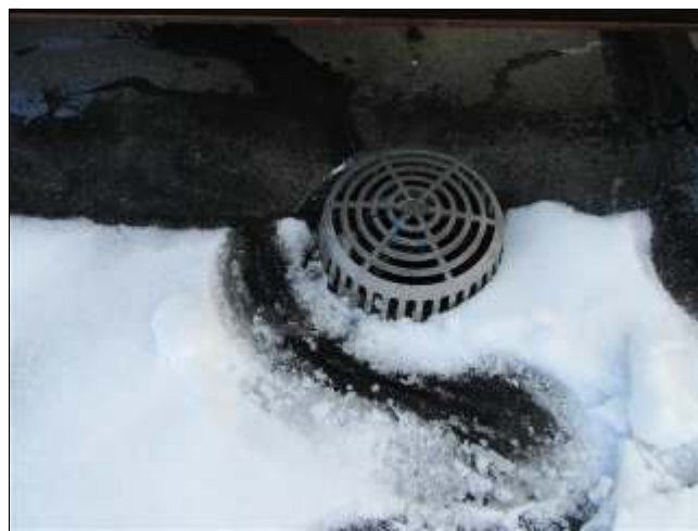
3.3 Item 4(Picture) Typical drain.
