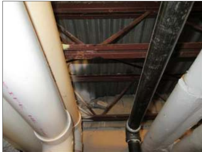
5.2 Item 2(Picture) Open web joists in good condition.
