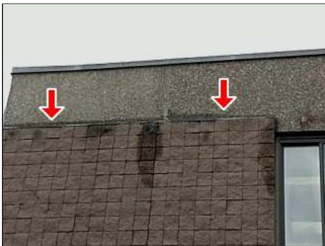
4.0 Item 1(Picture) Sealed joint.
