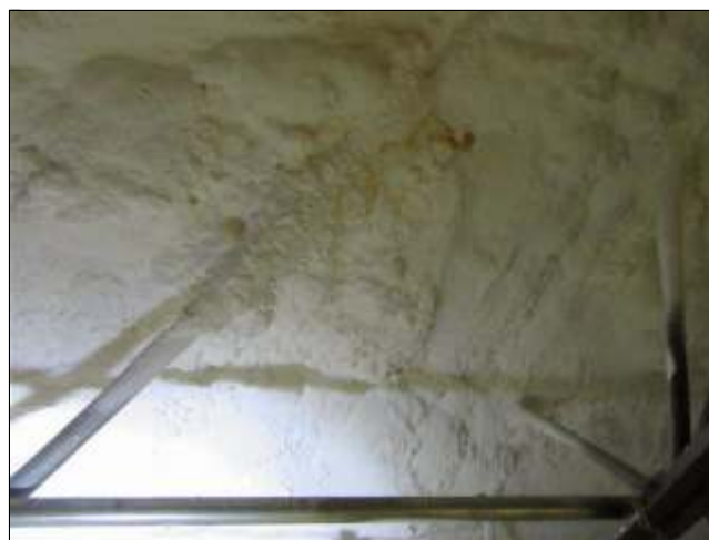
5.4 Item 2(Picture) Spray foam at perimeter.
