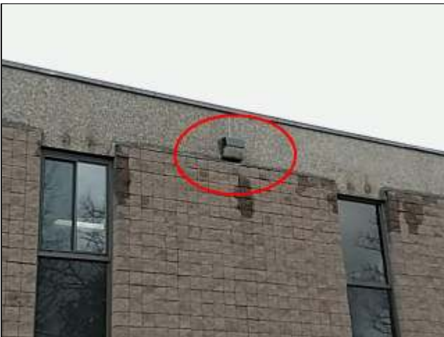
1.4 Item 1(Picture) Typical surface mounted light.
