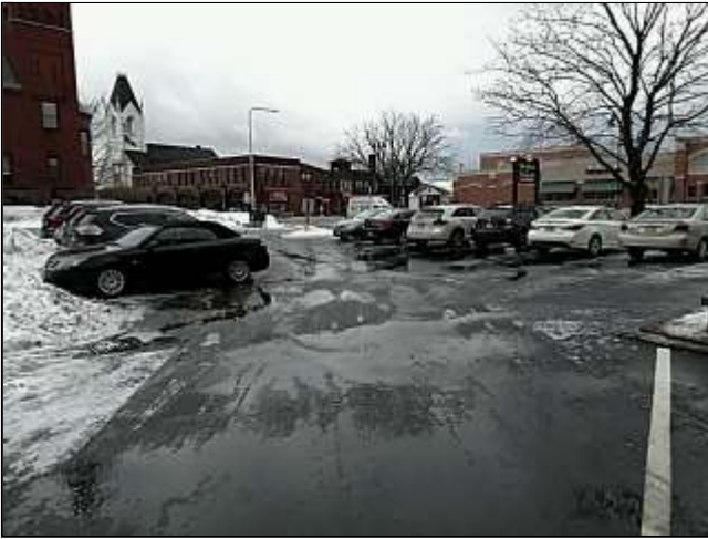
1.3 Item 5(Picture) View of rear parking lot.
