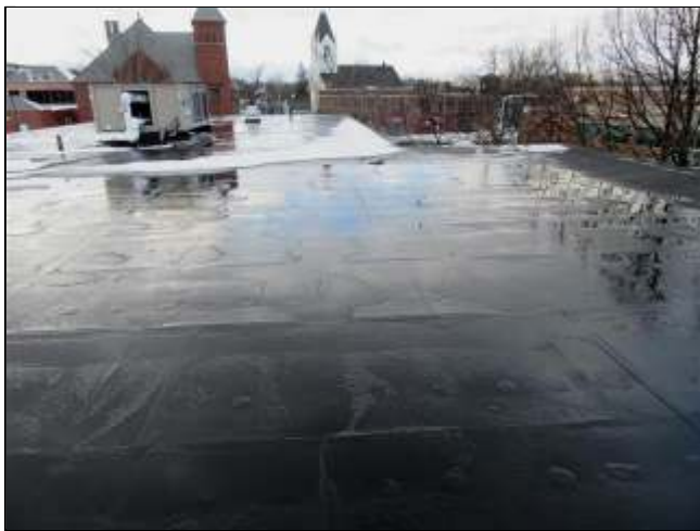
3.0 Item 1(Picture) View of roof.
