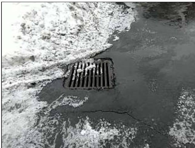
1.1 Item 3(Picture) Rear drain / functioning as intended.
