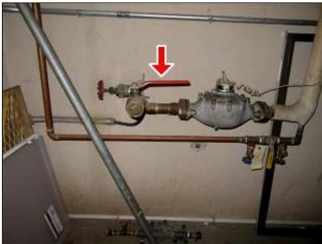
2.0 Item 1(Picture) Water main.
