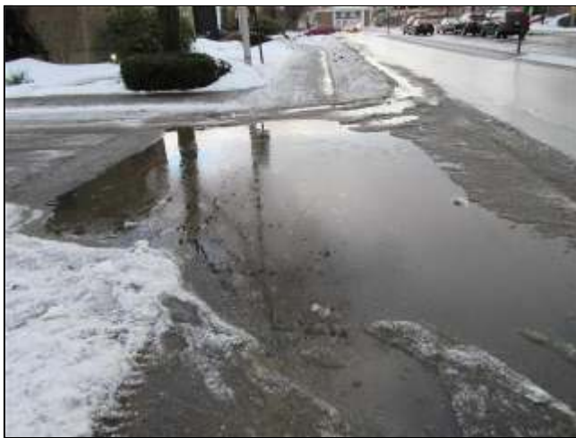
1.1 Item 1(Picture) Ponding/front entrance.
