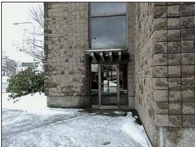
1.2 Item 1(Picture) Right front entrance.
