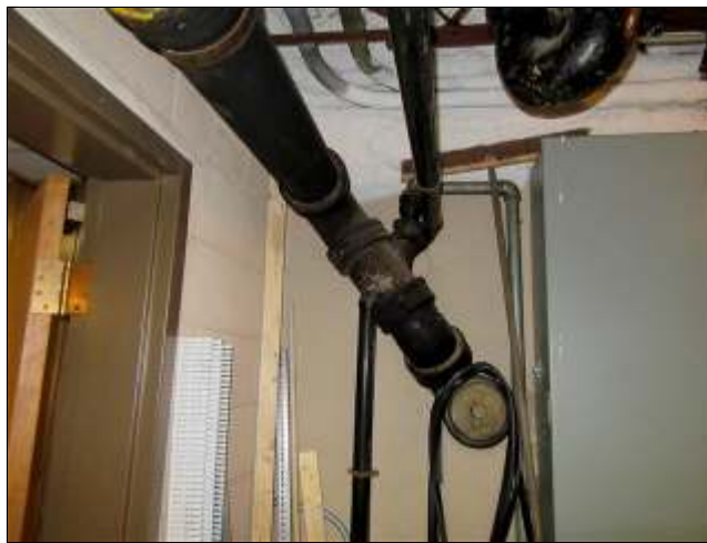
2.3 Item 2(Picture) Roof and sump pump drain/south side.
