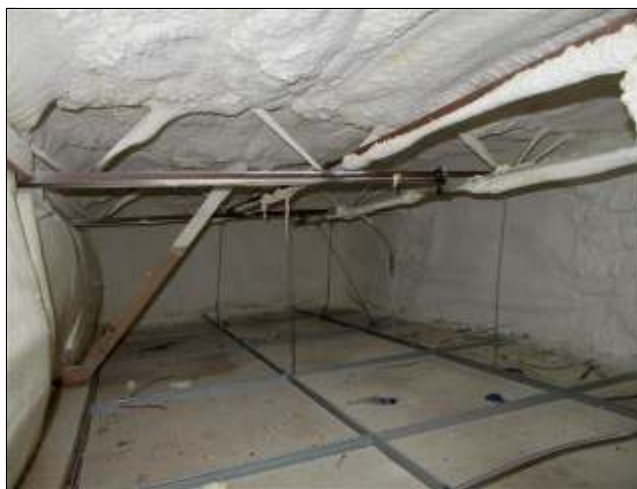
3.5 Item 4(Picture) Spray foam in good condition.
