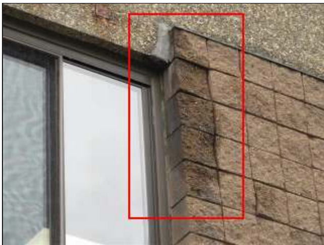
4.0 Item 5(Picture) Previous repairs.
