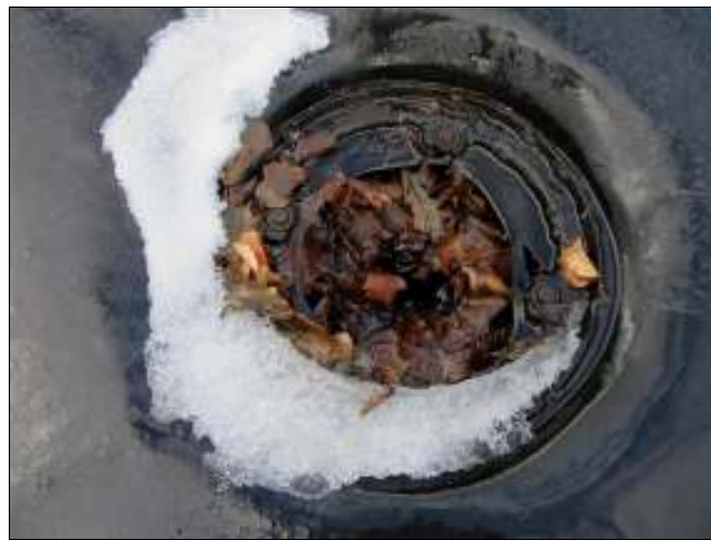
3.3 Item 2(Picture) Loose screen/debris.
