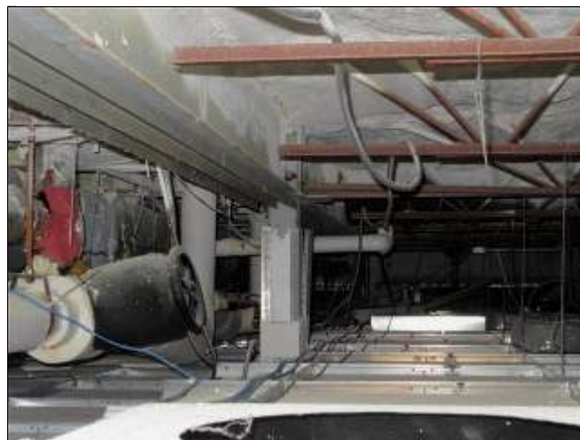
3.4 Item 2(Picture) Roof structure in good condition.
