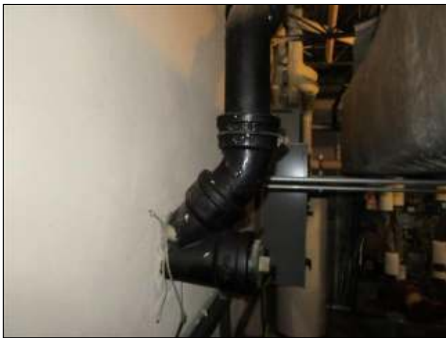
2.3 Item 1(Picture) Main sewer line/SW side.
