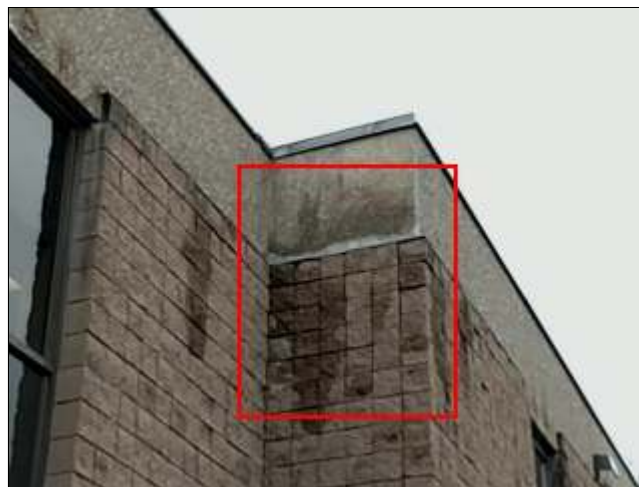
4.0 Item 2(Picture) Previous repairs.
