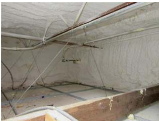
3.5 Item 3(Picture) View of insulation/roof hatch.
