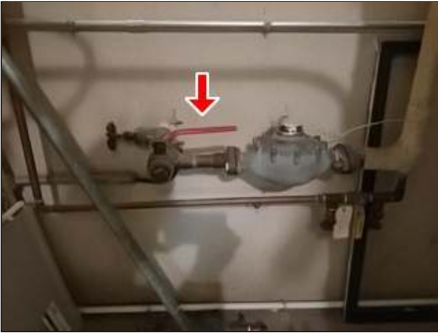
6.3 Item 1(Picture) Water main.
