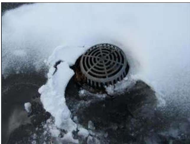
3.3 Item 3(Picture) Typical drain.
