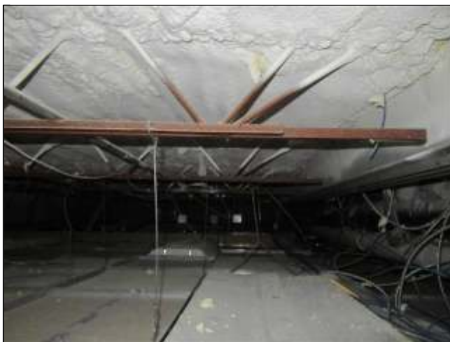
3.4 Item 1(Picture) View of roof structure.
