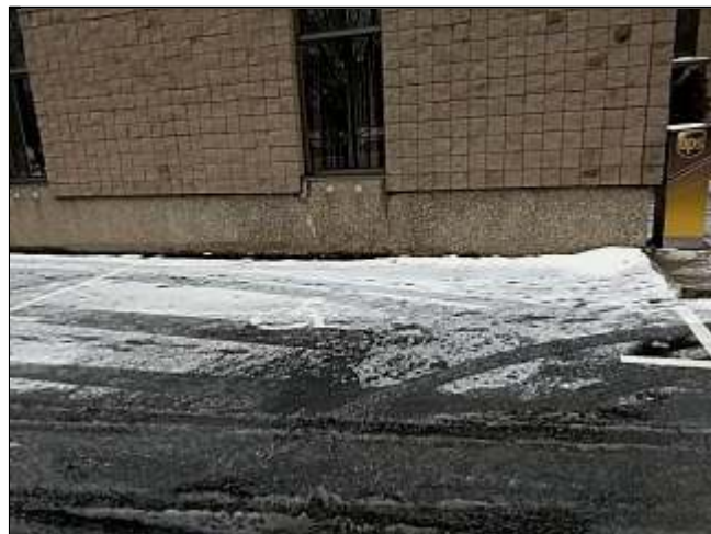
1.3 Item 4(Picture) No signage for designated handicap parking.
